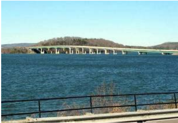
Bridge over Tennessee River and Guntersville Lake
